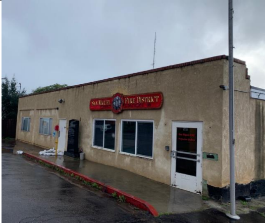
Photo of the Crest Station 18
