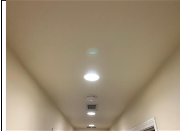
Photo of sample number 15, BDL Drywall Ceiling, Within Hallway
